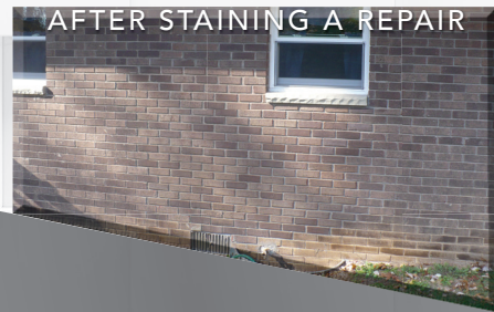
AFTER STAINING A REPAIR
